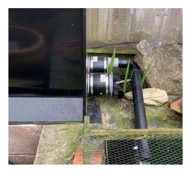
To Recap, maximum height water level should be when pumps are running is 254mm below filter top.
